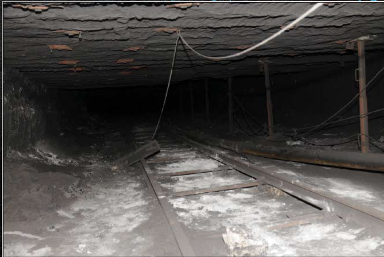
UBB Post-Explosion Photo Massey Internal Review Report - Figure 31
